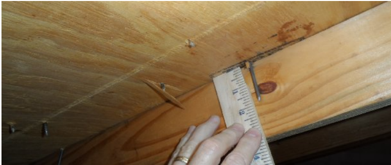
8d nails verified
