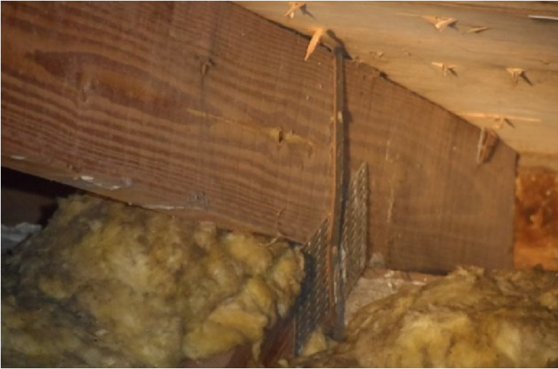
Single strap with 2 nails into the truss
