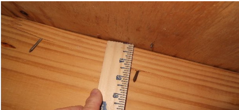
8d nails verified
