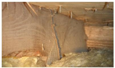
Single strap (clip) with at least 3 nails into the truss
