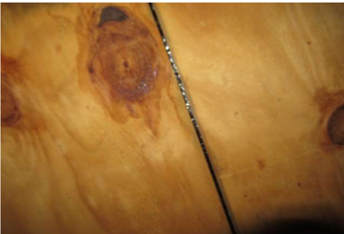
SWR installed under the tile
