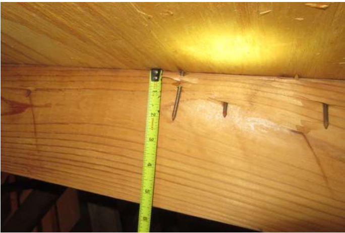
8d nails verified
