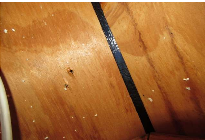
SWR installed under the tile
