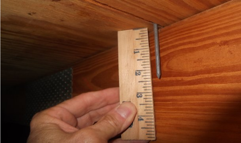
8d nails verified
